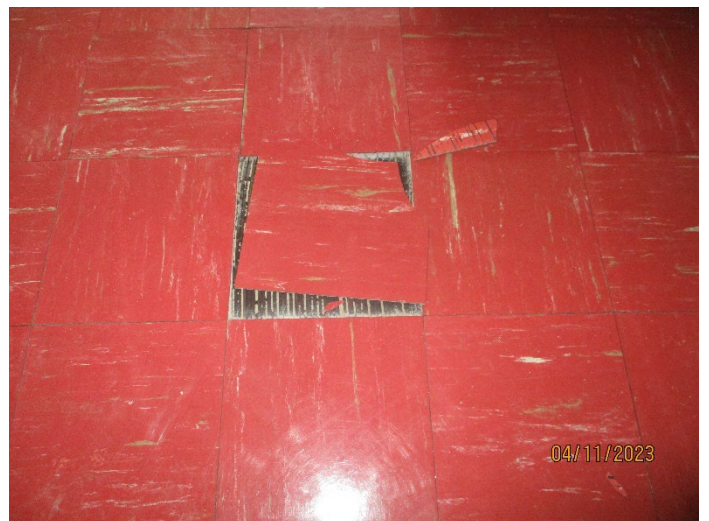
Photo 6 (April 11, 2023): ACM 9"x9" red floor tiles (sample set 053) located on the first floor of the 1968 addition.
