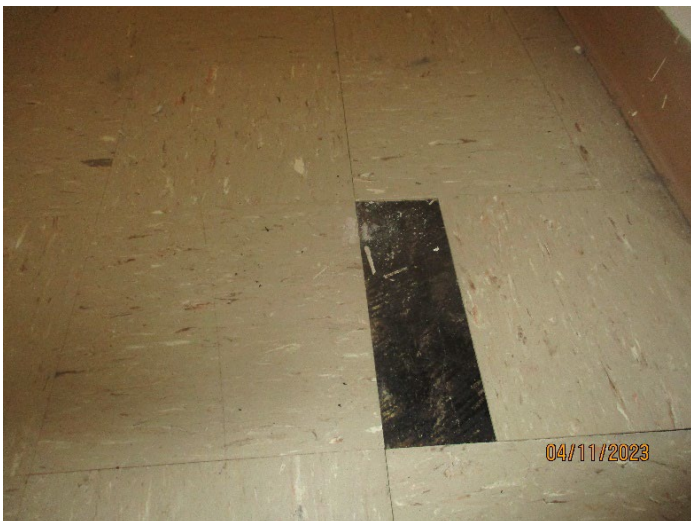
Photo 5 (April 11, 2023): ACM 9"x9" floor tiles (sample set 052) located on the second floor of the 1968 addition.
