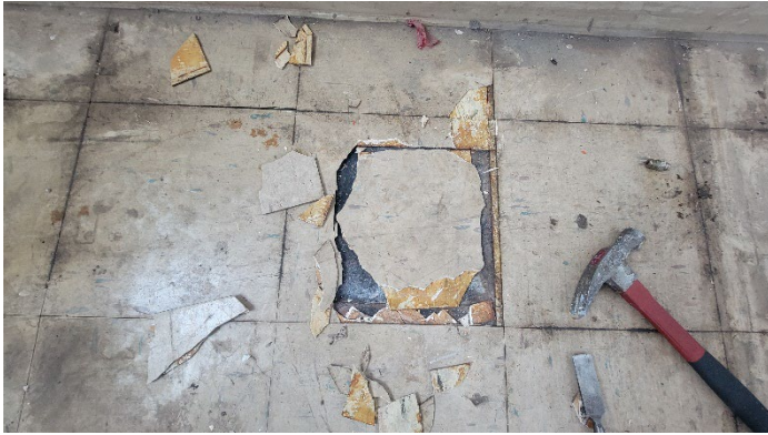
Photo 1 (April 6, 2023): Non-ACM 12"x12" floor tile and mastic (sample sets 008 and 009) over ACM 9"x9" floor tile (sample set 010) and associated mastic (sample set 011) located in the shop restroom.
