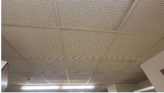
Photo 1 (April 6, 2023): PACM ceiling tiles located in the girl's locker room of the 1968 addition.
