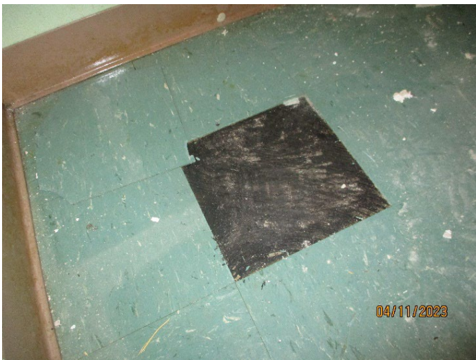
Photo 3 (April 11, 2023): ACM 9"x9" floor tile (sample set 049) and associated mastic (sample set 050) located in the second-floor band room closets in the 1968 addition.
