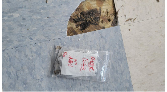
Photo 2 (April 7, 2023): ACM tan/black mastic (sample set 016ABC) beneath non-ACM 12"x12" floor tiles on the first and second floors of the 1968 addition.
